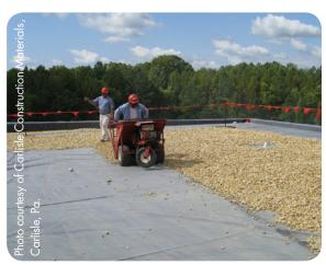
Roofing professionals spread ballast and level out the stones to ensure even coverage.
