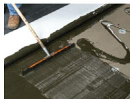
An asphalt-modified polyether, one-sided, wet lay-in adhesive designed to adhere to VersiFleece AC membranes and Versico's modified base sheet.
