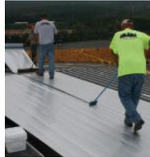
A 15-mil composite reinforced aluminum-coated poly with a self-adhering SBS. Used as an air and vapor barrier direct to metal decking. Meets UL 1256 and FM 4470 internal fire ratings. Reinforced aluminum-coated poly stands up to the toughest roof traffic. This product's self-healing characteristics allow for fastening penetration while maintaining IECC air leakage requirements of 0.04 cfm.
