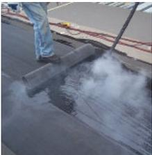
A 90-mil SBS-modified asphalt base sheet. Can be used in multi-ply roofing systems as an air and vapor barrier, or as a temporary roof for up to 60 days. This product is fiberglass-reinforced and meets or exceeds requirements of ASTM 6363 Type 1. When used as an air and vapor barrier, suitable substrates include concrete (primer required), DensDeck Prime, and SECUROCK.
