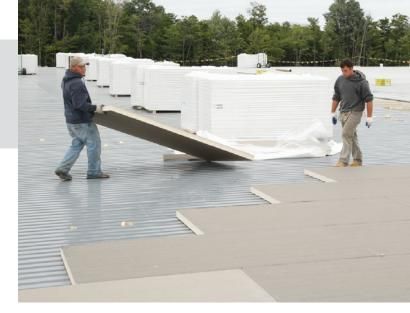
(LBC) "Red List Free" rigid roof insulation panel composed of a closed-cell polyisocyanurate
