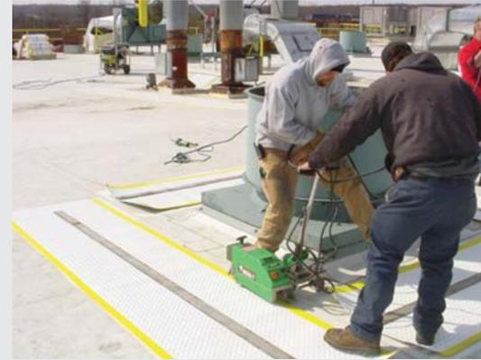
4. When walkways are to be installed perpendicular to field splices, adjust walkway length to provide a 4"–6" minimum gap at field splices. Because the attachment of the walkway to the membrane is permanent, this will allow access to the field seams.
