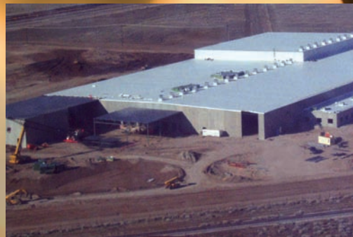
New Versico Manufacturing Plant, Tooele, Utah
