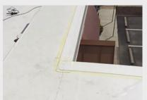
5. Install PVC PS Cover Strip as soon as the PVC Step 2 Primer or Low-VOC PVC Step 2 Primer flashes off to minimize the potential for dust contamination and to promote adhesion in colder weather. Peel off 10"-12" (250-300 mm) of the protective release liner from the PVC PS Cover Strip. Position the flashing and press down using firm, even hand pressure across the entire area. Continue this process until the full area to be flashed is completed.
