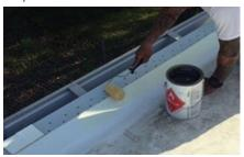
4. VERY IMPORTANT: Wherever the PVC Pressure-Sensitive Cover Strip is to be overlapped (at any overlaps, corners and end laps), be sure to apply Low-VOC Step 1 Activator to the overlap area of the previously installed PVC PS Cover Strip before applying the PVC Step 2 Primer or Low-VOC PVC Step 2 Primer. This applies to all inside and outside corners and end laps.
