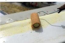
Roller-apply PVC Step 2 Primer or Low-VOC PVC Step 2 Primer to the area already covered by the PVC Step 1 Activator and to the previously cleaned metal to be flashed. The properly primed area will be uniform in color, without streaks, and free of globs or puddles.
