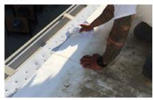
Use a 3"-wide, short nap-length paint roller to apply PVC Step 1 Activator. Only apply activator to the area where PVC PS Cover Strip will be applied. The properly activated area will be uniform in color, without streaks, and free of globs or puddles. Let dry. DO NOT APPLY PVC STEP 1 ACTIVATOR TO ANY OTHER SURFACES EXCEPT THE PVC OR KEE HP MEMBRANE TO BE COVERED BY THE PVC STEP 2 PRIMER AND THE PVC PS COVER STRIP.
