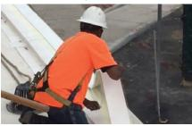
To achieve proper adhesion of the PVC PS Cover Strip when jobsite temperatures fall below 40°F (5°C), heat the cleaned and primed area of the membrane with a hot-air gun as the flashing is applied and pressed into place.
